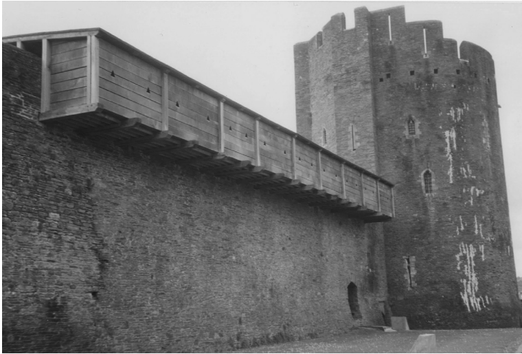
Figure 1.5 Hoarding at Caerphilly Castle. The defences projecting from the wall made it very difficult to start mining at the base or mounting ladders. Author's photograph.
